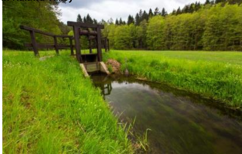
Przymuszewo FD – small water gates-culvert in Kulawa Valley
